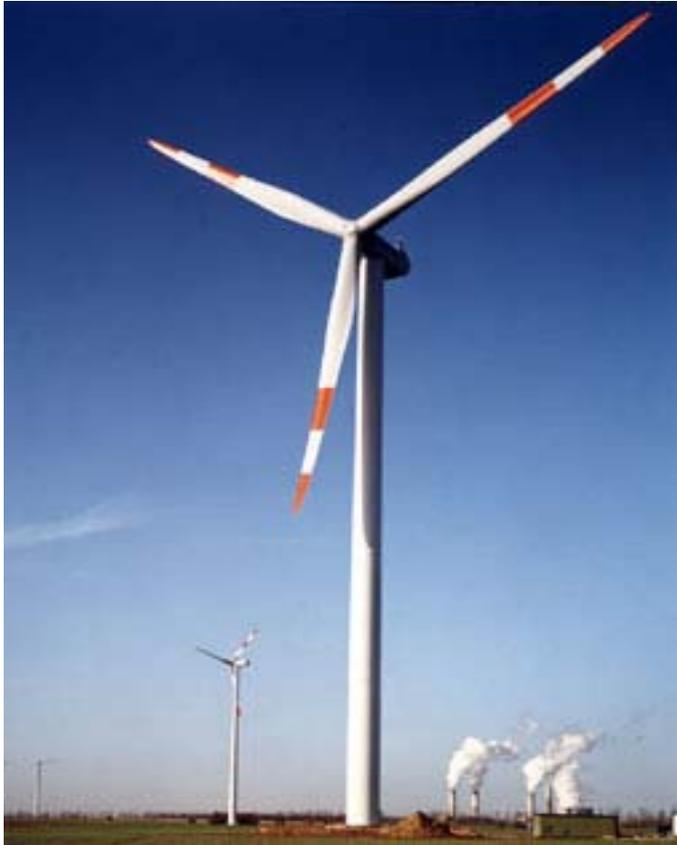
*Prototype of 80 m tall Nordex 2,5 MW wind turbine located in Grevenbroich, Germany
